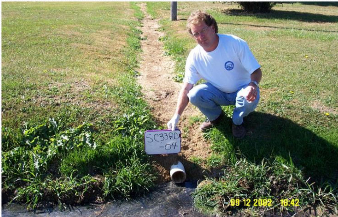
Cheater pipes to a ditch
