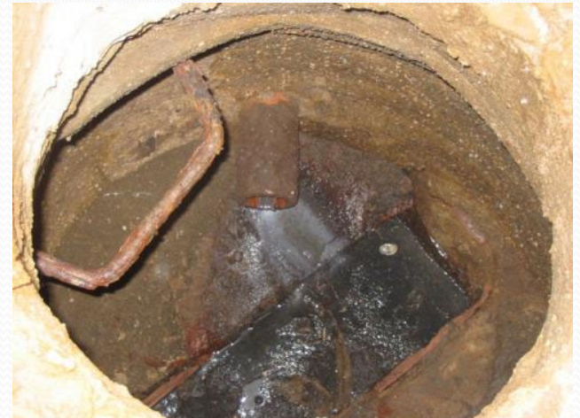
Gray/black staining in a storm sewer
