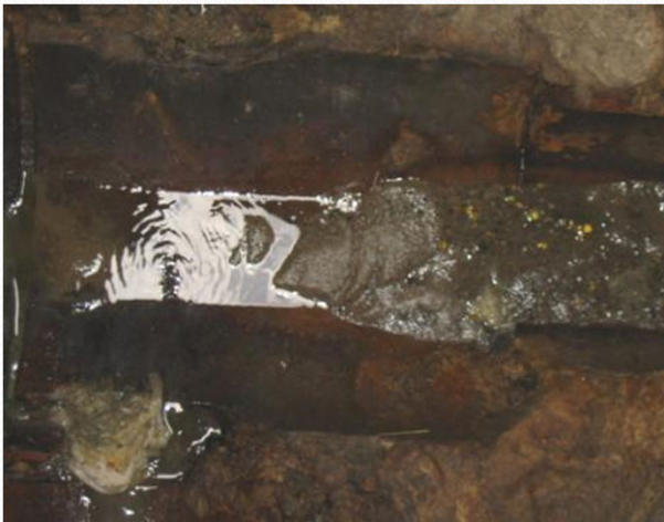
Sanitary debris in a storm sewer
