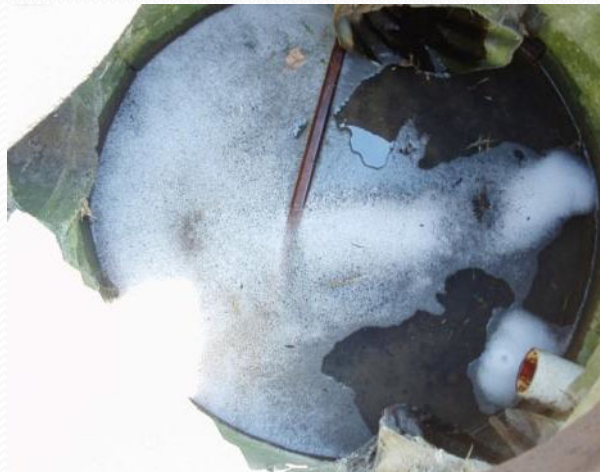
Soap suds in a storm sewer
